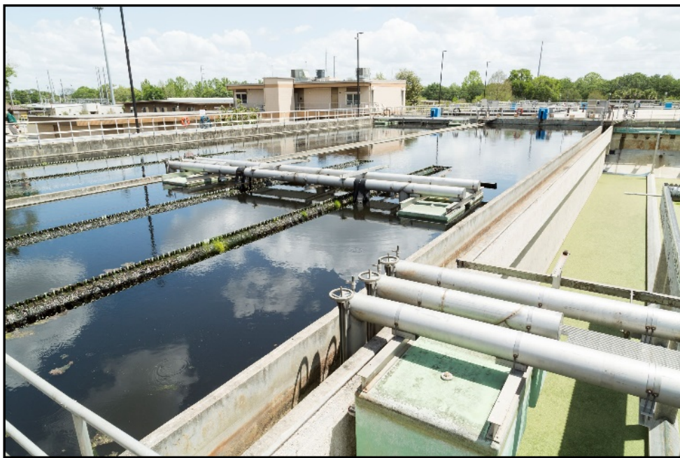
Figure 1. Altamonte Springs Regional Water Reclamation Facility
